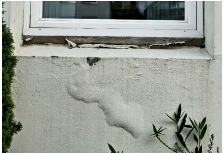
Pictured above: Water pockets have been pooling behind the paint on City Hall's exterior
