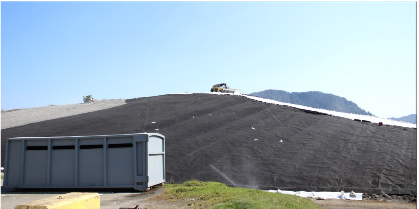
Pictured above— Major works to cap the existing landfill cell occurred in 2024
